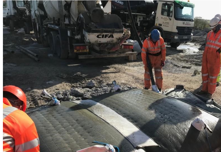
Concrete mattress placement by TMS on Isle of Man in 2019
