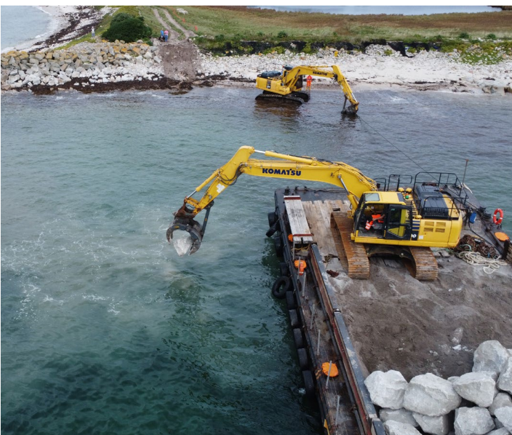
Rock armour placement, Isles of Scilly TMS Maritime 2024
