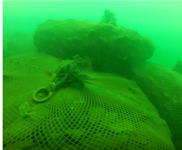
Installed rock bags underwater by TMS on Isle of Man in 2019
