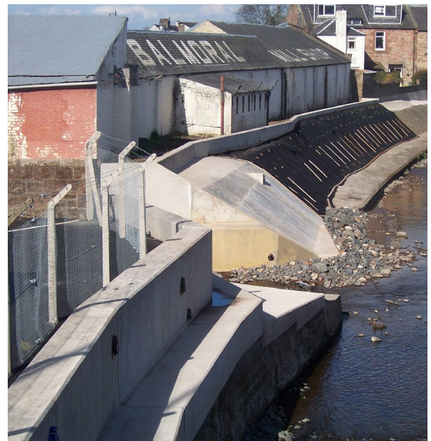
Concrete revetment on River Irvine, Scotland 2007
