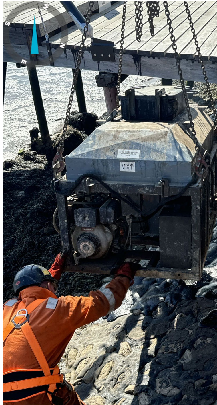
Bituminous Asphaltic Grouted Rip Rap by HEP 2025
