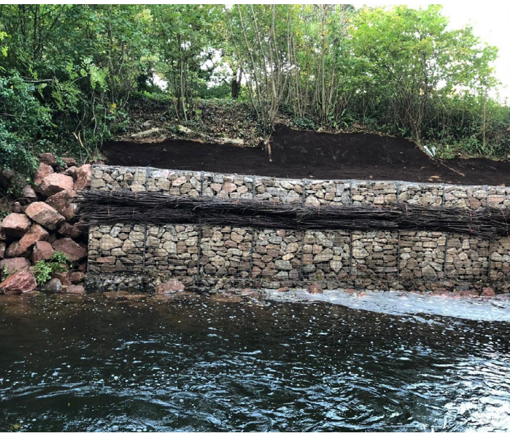
Gabion wall installed in Newton St. Cyres by TMS in 2018
