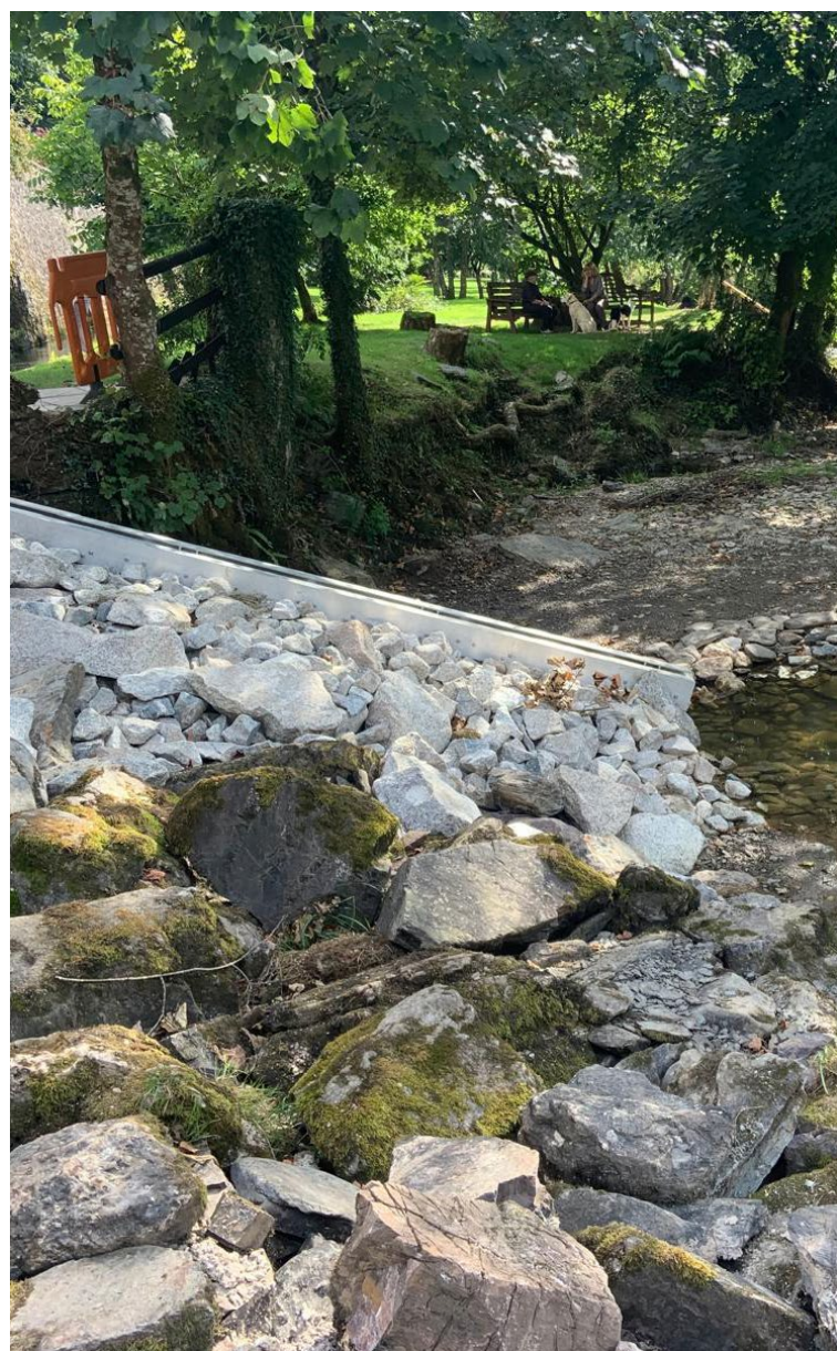
Riprap weir protection installed in Bridge Town by TMS
