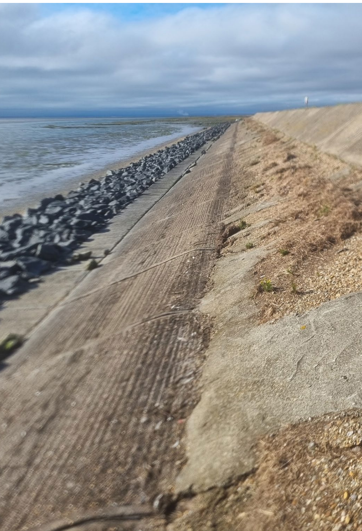
Concrete Revetment, HEP site visit
