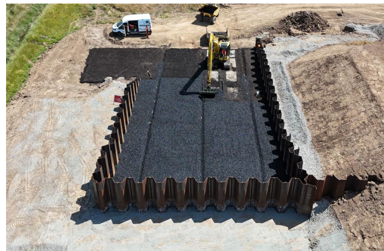
OSA Pump Discharge Channels, Winestead 2025
