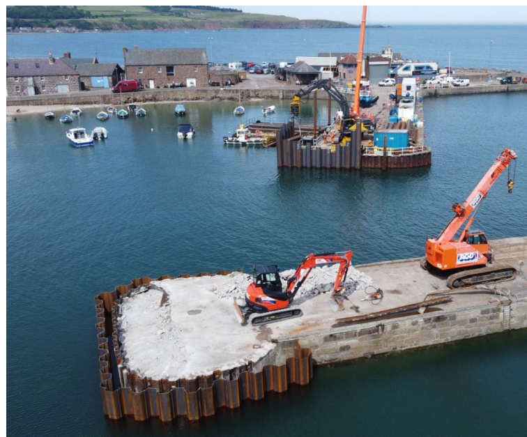
Sheet Pile Installation in Stonehaven by TMS 2022
