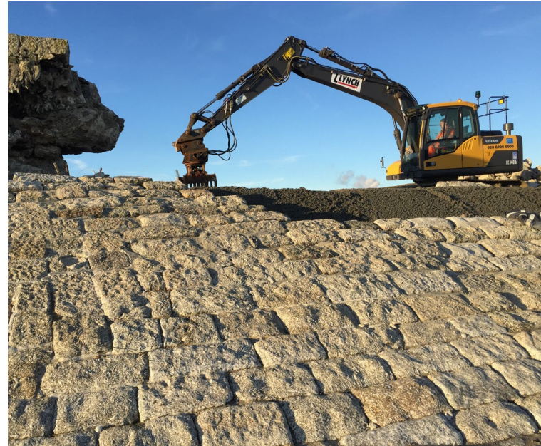
Stone block revetment in Par Harbour by TMS
