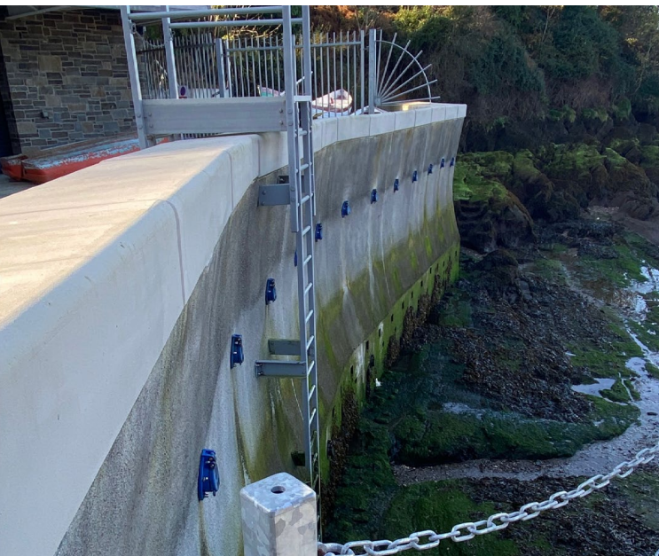
In-situ concrete sea wall in Ifracombe
