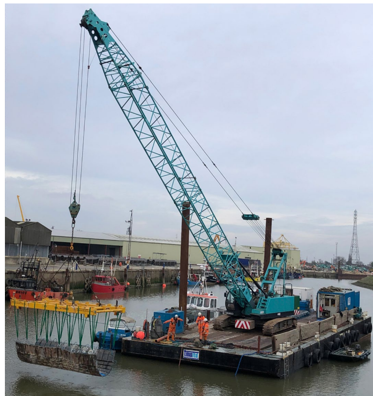
Articulated Concrete Blocks installation by TMS Boston Barrier 2019
