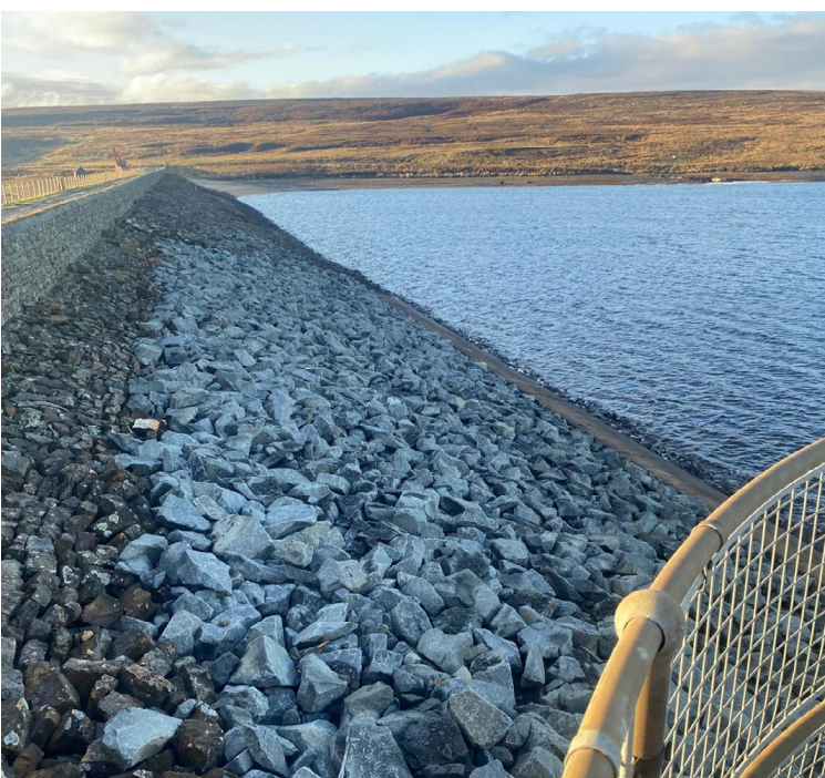
Riprap revetment installed in Durham by HEP
