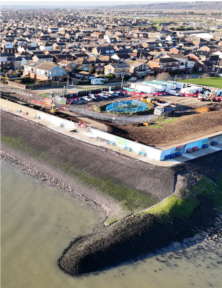
OSA Revetment by HEP, Canvey Island 2023
