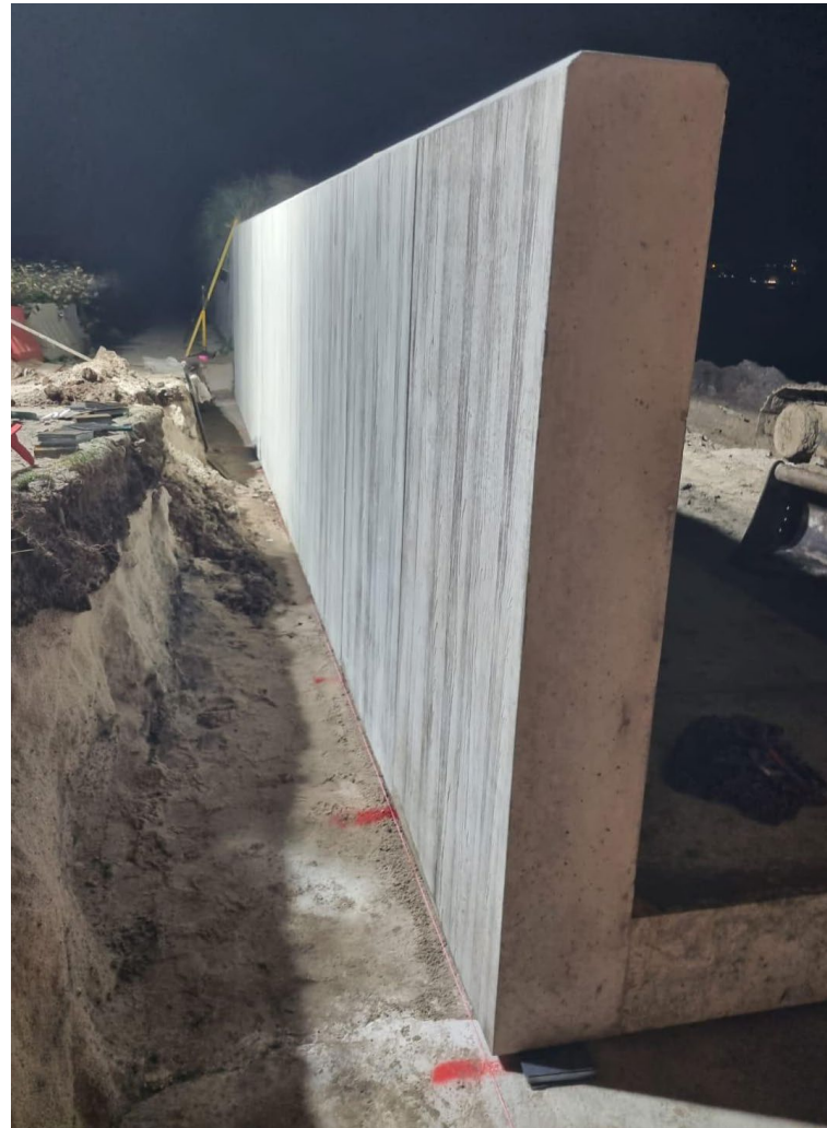
Installation of pre-cast concrete sea wall on Isle of Mann 2019 by TMS
