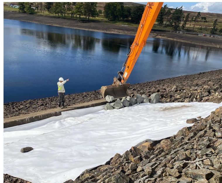
Rock Armour placement, Waskerly Reservoir 2024
