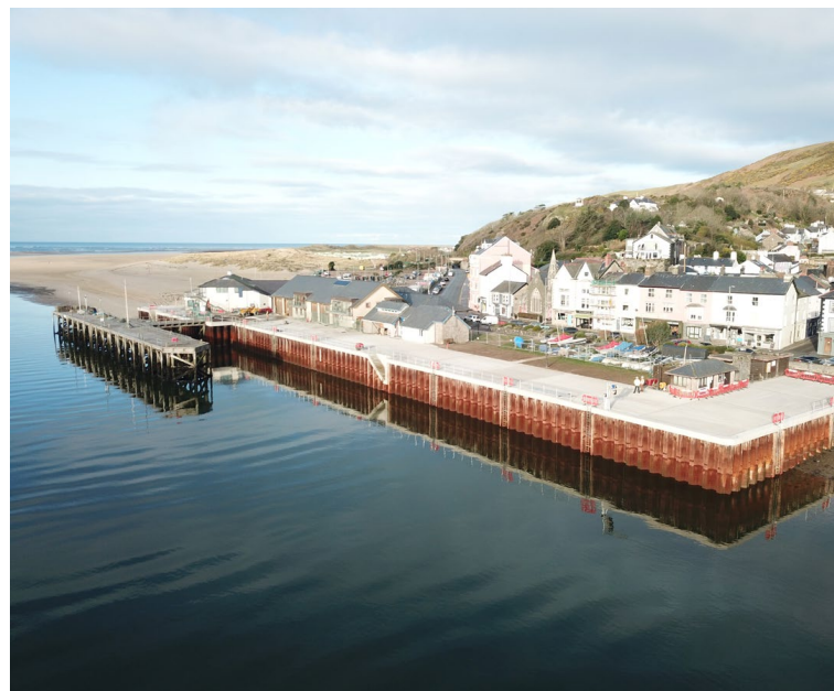
Sheet Pile Installation in Aberdyfi by TMS in 2022
