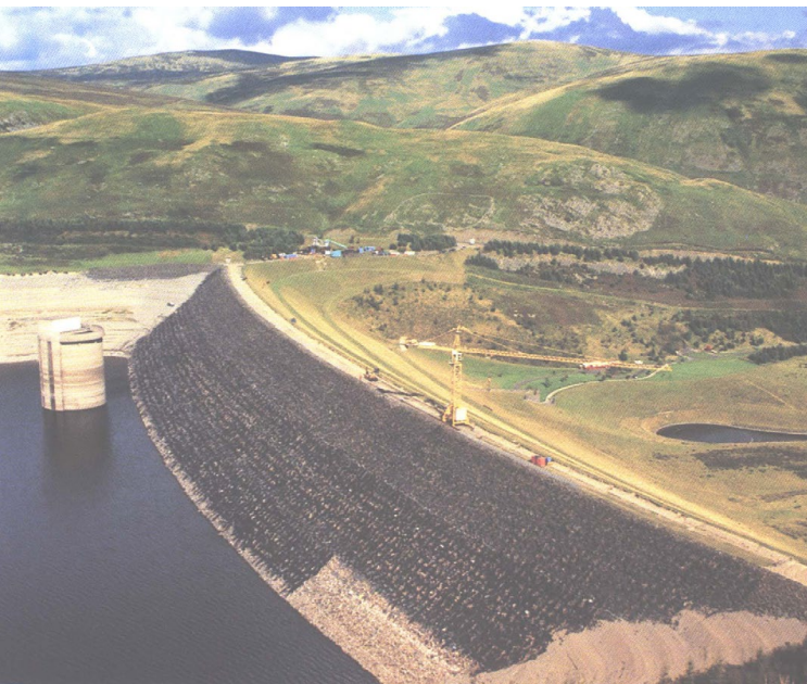
Bituminous Asphaltic Grouted Rock on Megget Dam by HEP 1997/1998
