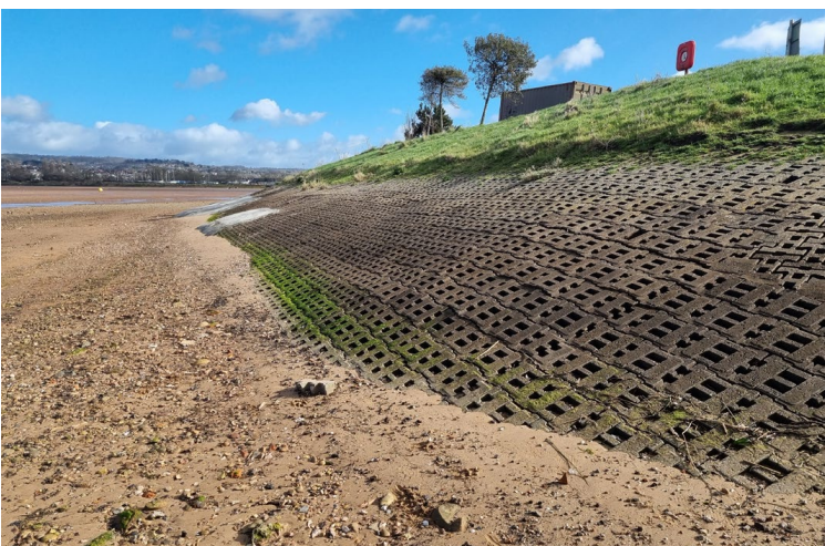
Articulated concrete block revetment
