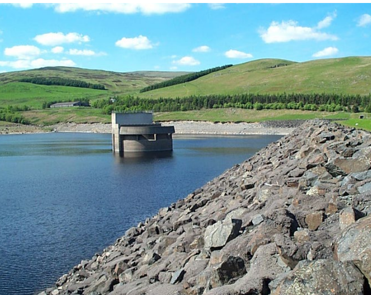
Megget Dam, Scotland. An HEP project
