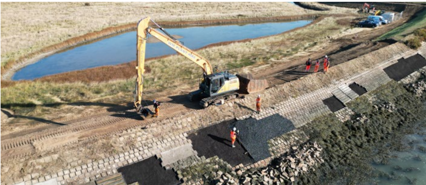
HEP repairing sections of a concrete block revetment, Essex
