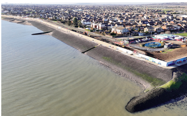
Part of 3km coastal revetment completed on Canvey Island
