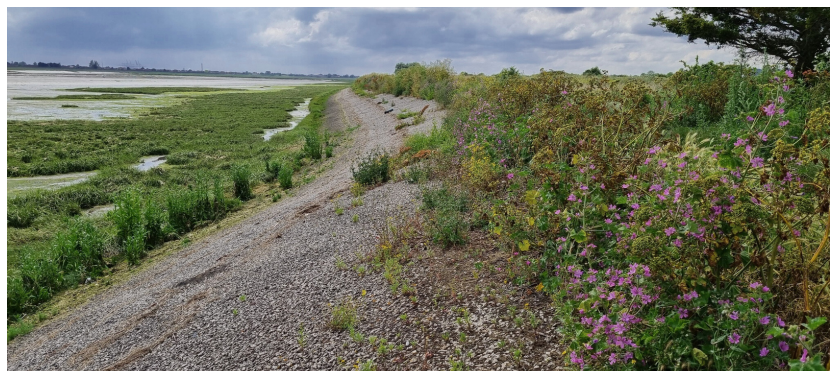
OSA revetment 19 years after installation on Two Tree Island
