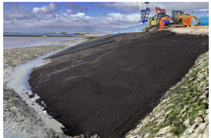
LSA used overlaid on existing revetment tying into groyne prior to OSA layer
