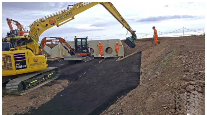
LSA shaped to form channels and embankments for pump outfalls
