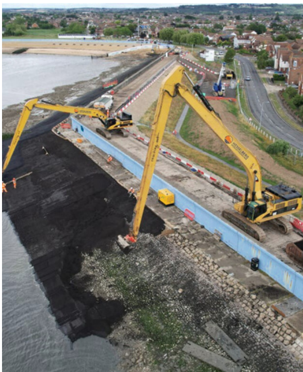
LSA being placed as void filler and filter layer
