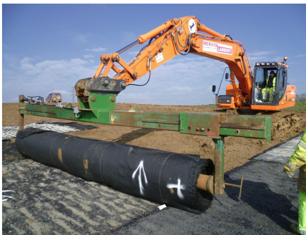
Installation of Geomat DM20 using purpose built frame
