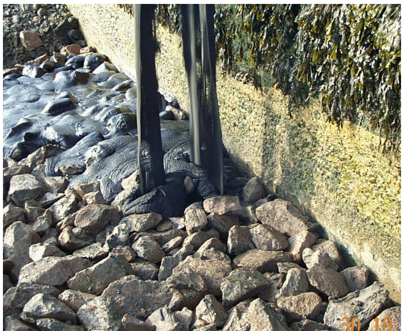
Full depth grouting to gabion stone
