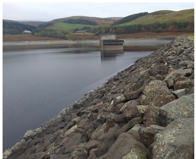
Megget Dam – pattern grouted in 1997-98, no maintenance needed – photo taken Oct 2025
